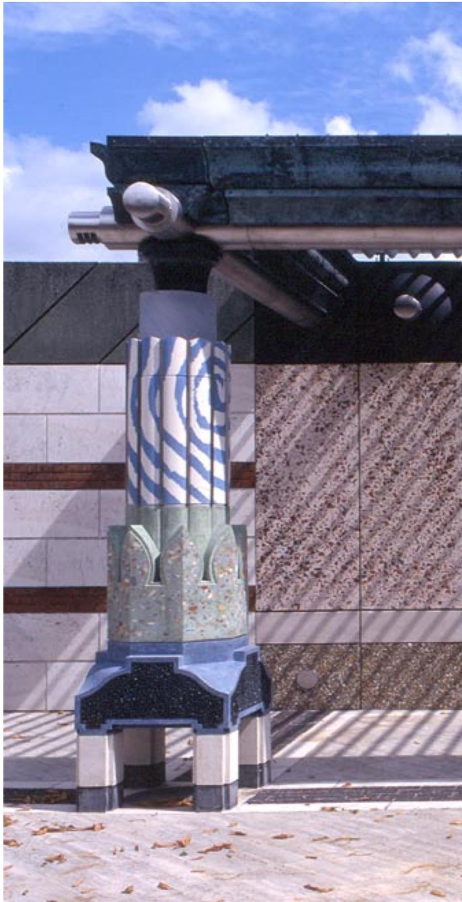
*Finished before January 1.1.2000 this Millenium Pavilion has a fabric canopy that extends forward out of the 'cavetto' or 'scotia' (meaning darkness and death) moulding of its post-patinated copper entablature. Its roof is of louvres that turn to open to the sun. Each louvre has a gutter that forbids drips when opened after rain.*
